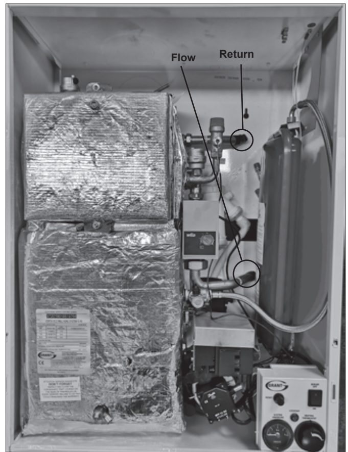
Figure 5-2: System boiler flow and return connections
